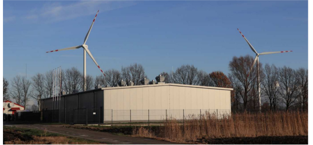
Poland's largest hybrid battery energy storage system. Source: Sumitomo Mitsui Banking Corporation.
