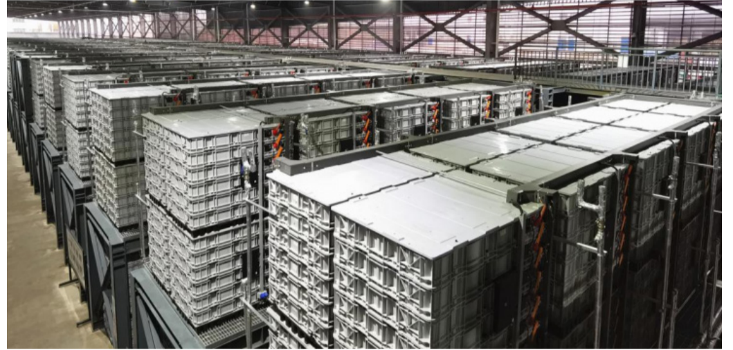
LDES system made of advanced lead-carbon batteries in Huzhou, China. Source: China Daily
