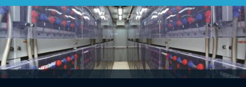
The battery is operated at partial state-ofcharge so that it can accept and deliver charge at all times. The lead-carbon technology used was developed in partnership with ALABC. These REX Carbon cells have a projected calendar life of 15 years and an extended cycle life in shallow cycle service.
