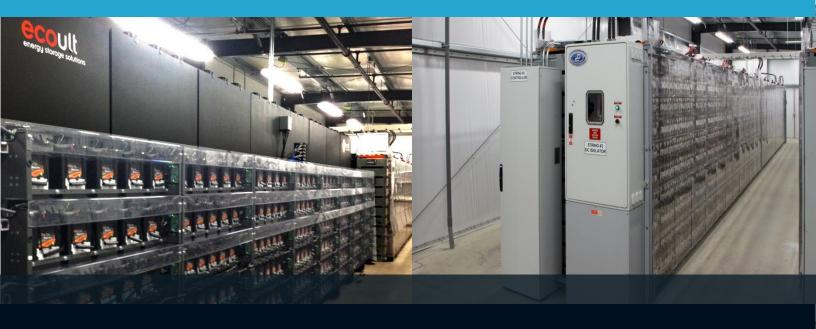
For frequency regulation services, the batteries roam in approximately 40% Partial State-of-Charge band. The system implements an application that follows the PJM signal and maintains the State-of-Charge (see below).
