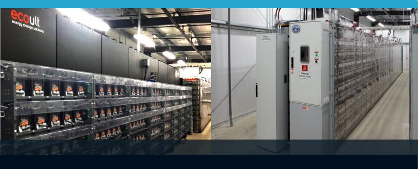
For frequency regulation services, the batteries roam in approximately 40% Partial State-of-Charge band. Ecoult implements an application that follows the PJM signal and maintains the State-of-Charge (see below).
