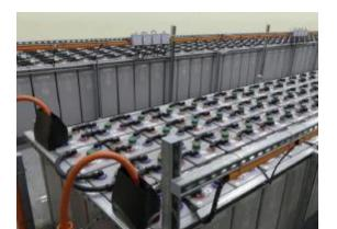
The project began in 2016 and was completed in 2017. Nuvation Energy installed a NuvationBMS™ High-Voltage Battery Management System that would provide precise State of Charge (SOC) information to the Siemens power conversion systems (PCS) to help manage the charge and discharge process. The BMS also provides remote access to battery performance data.
